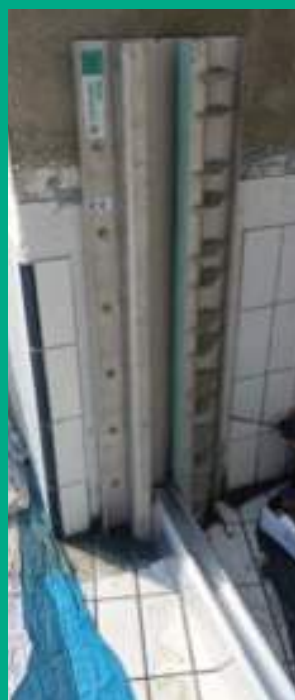
After installation – HydroBeam stoplog frame system
