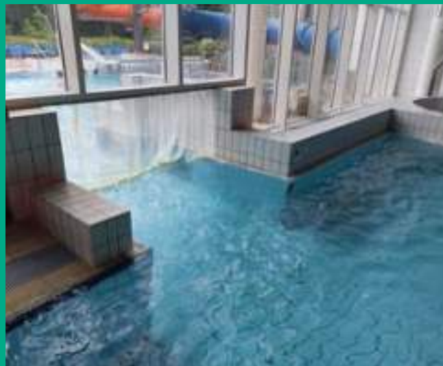
View of the indoor pool before installation
