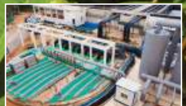
Odour Control system in Fathe Nagar
